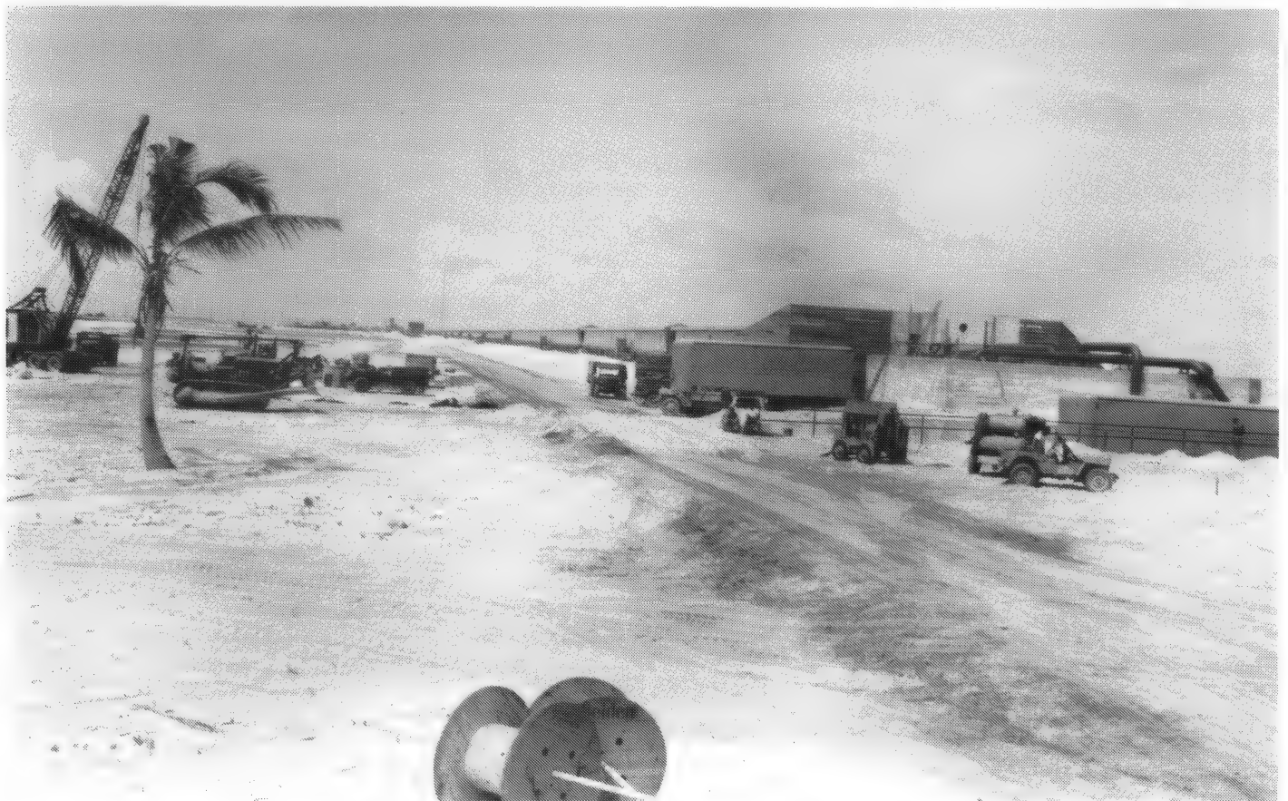
FIGURE 5-28. KRAUSE-OGLE HELIUM BOX FROM MIKE CAB TO STATION 200
